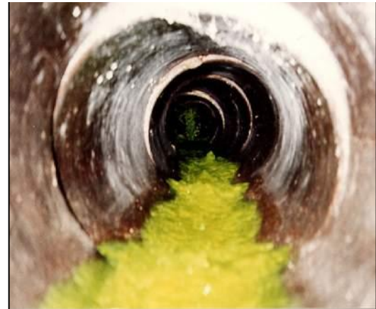
FIGURE 1.3.4 VIEW INSIDE SEWER PIPE FOR DYE TESTING
