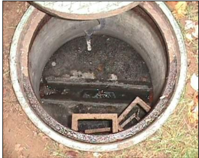
FIGURE 1.3.2 VIEW INSIDE A MANHOLE
