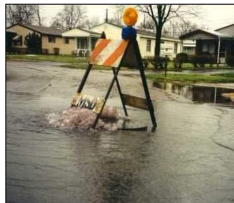
FIGURE 1.3.5 OVERFLOW DURING WET WEATHER
