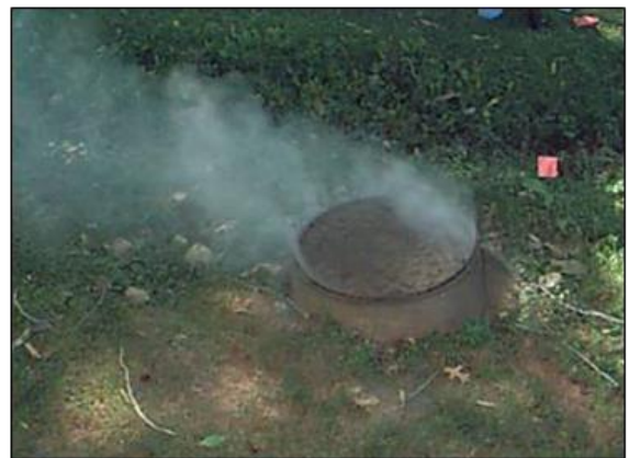
Figure 1.3.1 Smoke Indicating an Inflow Source at Manhole
