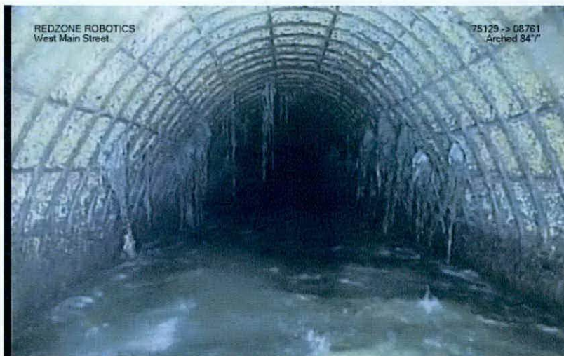
Video and laser inspection show concrete worn away and exposed rebar due to corrosion from sewer gases, particularly between 4 th and 7 th streets along West Main St.
