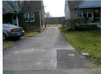
Private Property Sewer - Complete
