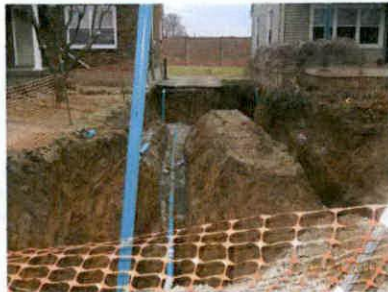
Private Property Sewer - During Installation
