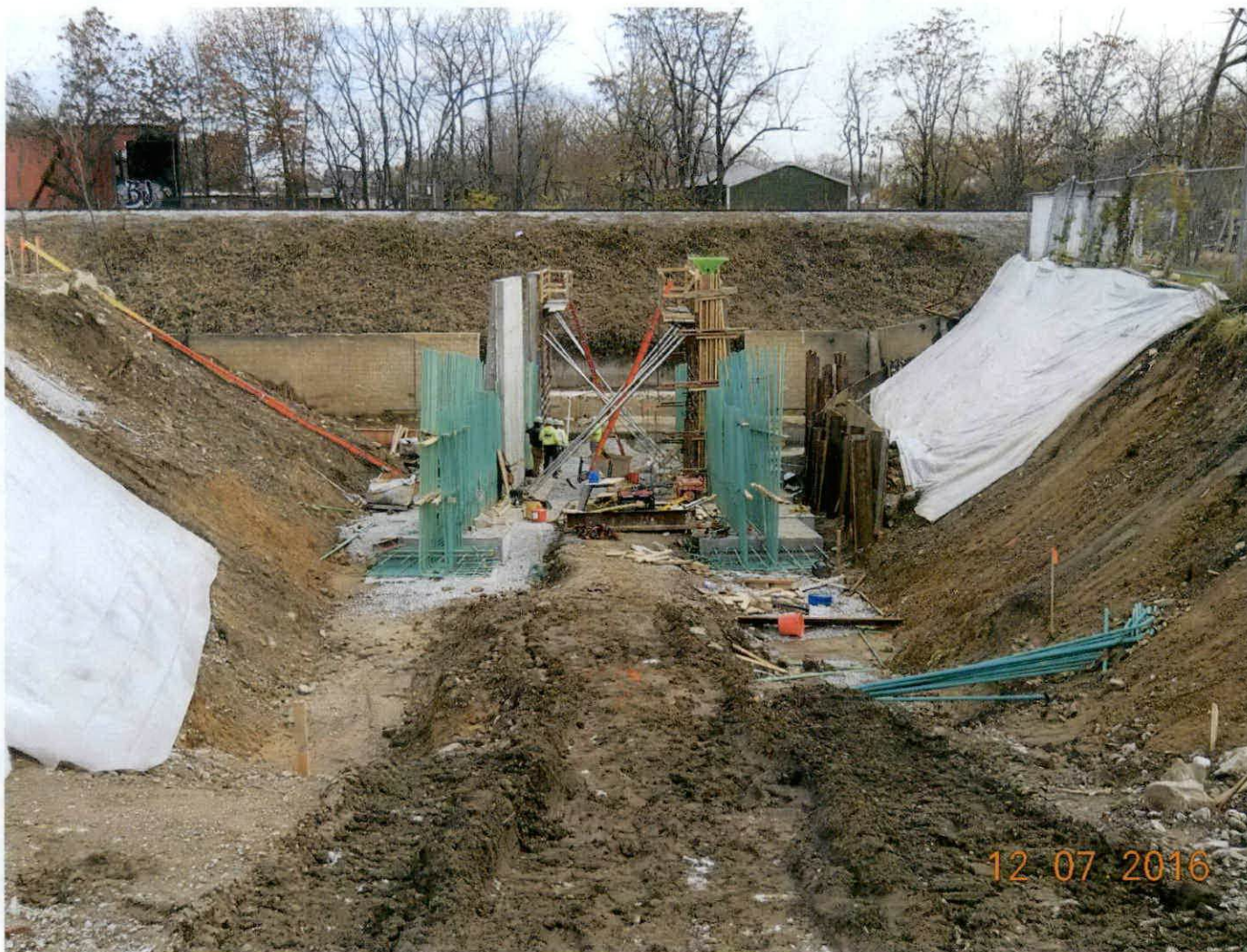
Logan Street Access Ramp
