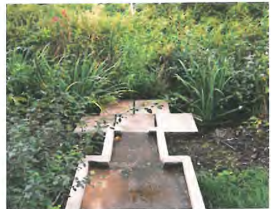
Rain gardens help capture rainwater and prevent overflows.
