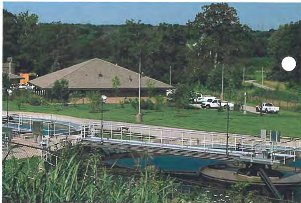
Floyds Fork Water Quality Treatment Center
