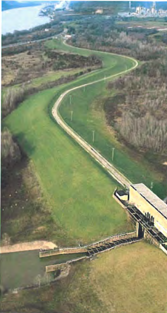
Pond Creek Flood Pumping Station
