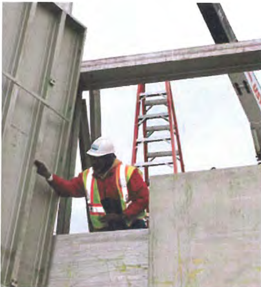
Ohio River flood gate installation
