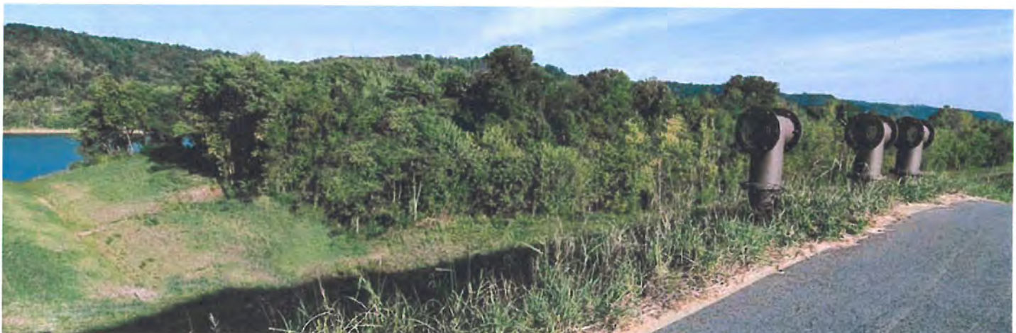
Ohio River levee in southwest Louisville Metro
