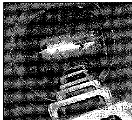
MSD cleans a catch basin with a clamshell bucket.
