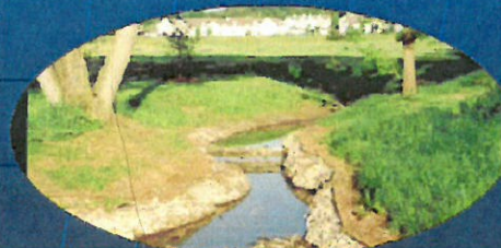
9 Springs Creek - Fitchburg, WI
