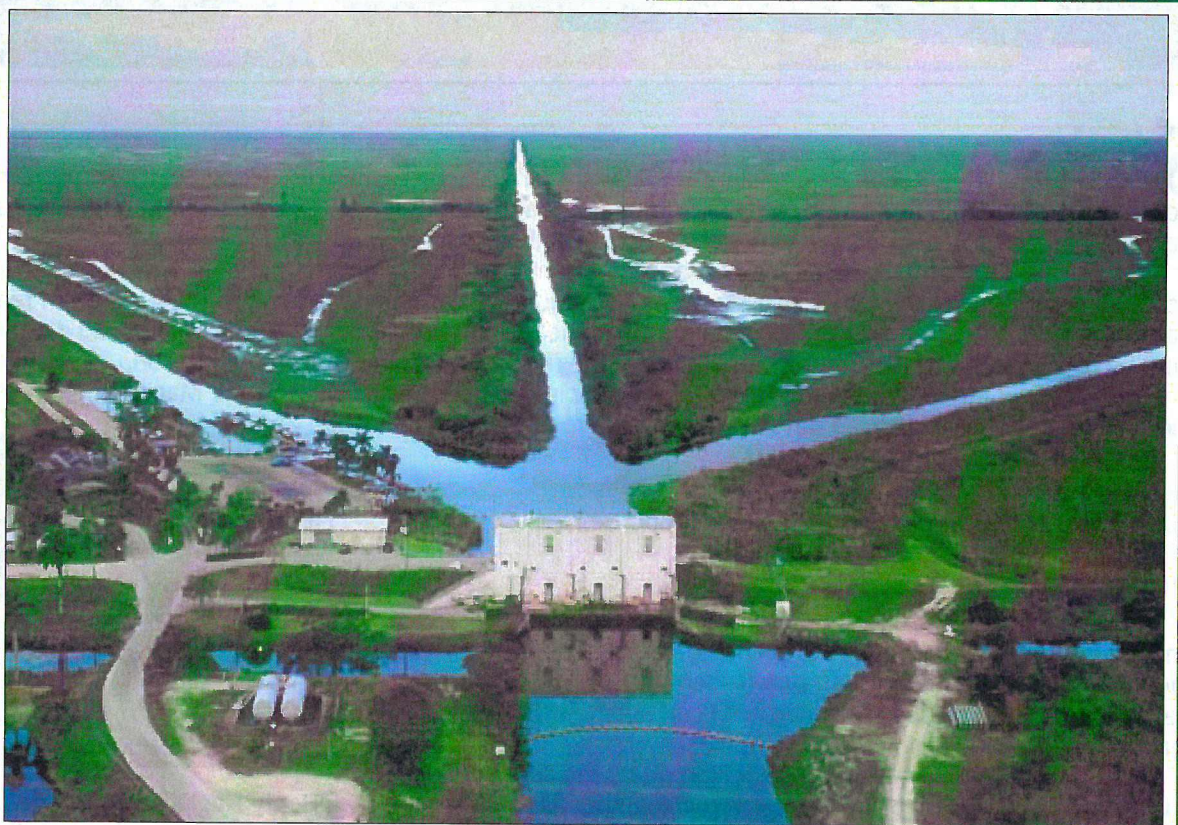
The S-9 pumping station, located in Broward County, is the primary discharge structure for the C-11 West Basin, one of the urban tributary basins discharging stormwater runoff into the Everglades Protection Area.
