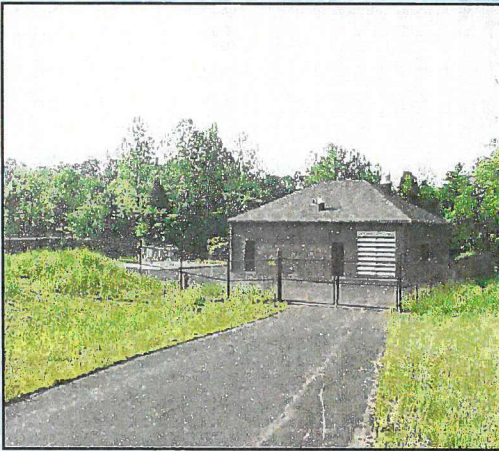
Long Run Pump Station
