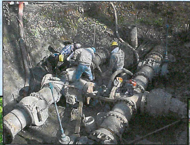
Ohio River Force Main Valve Impvts
