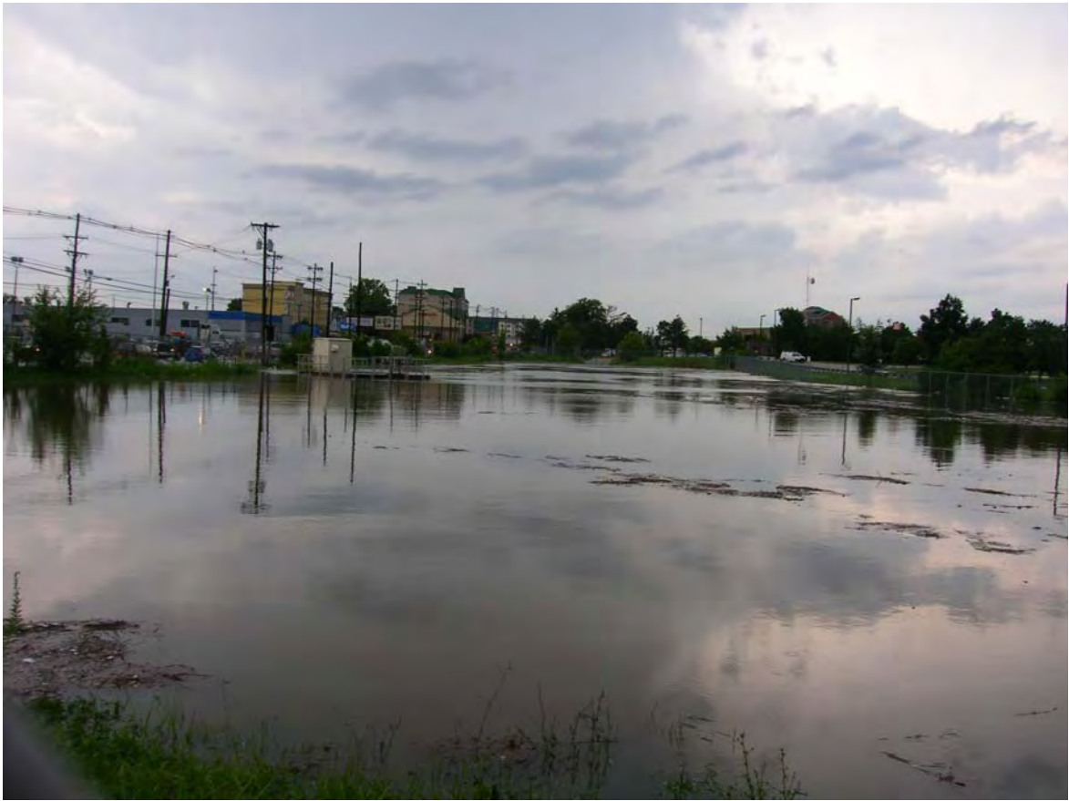
Fairgrounds Flood Control Basin.
