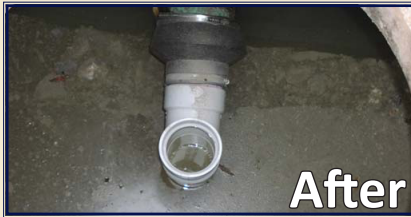
Same Grease Trap After Repairs and Cleaning
