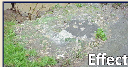
Sanitary Sewer Overflow Caused by Grease Accumulation
